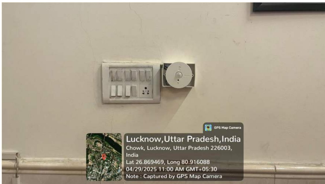
Sensor based Lights in the Administrative building room
